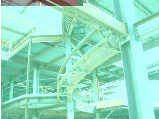
A large circular atrium is located on the south side of the office space. The atrium is 92 feet in diameter and extends one story below and two stories above grade. At the base a water feature was installed by a specialty contractor. Openings through the main and second floors provide uninterrupted views of the water feature and skylights. At the main and second floors the atrium is encircled with a 10 foot wide catwalk supported off the perimeter columns with knee braces.
