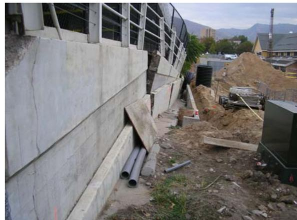
As seen in the above photo, the contractor placed a trench too close to a lateral earth retaining wall which resulted in a collapse of the wall.
