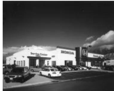
Curved beams at the front elevation are one of the required design features Ensign accommodated at the new Honda dealership facility, located on 1200 S. in Orem. Ensign has also designed the West Valley Dodge dealership, and is currently working on Toyota of Provo. All three dealerships are type II construction, with boundary collector elements transferring lateral loads to reinforced masonry piers.
