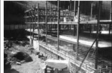
Ensign provided the design and detailing of the exterior panel system for this nine-story condominium and retail space, located at Big Sky Resort. The design requirements included seismic zone 4, 80 MPH Exp. "C" wind load, and 165 psf roof snow load, 100% in combination with seismic loading. The project is scheduled for completion late this year, with most of the exterior
