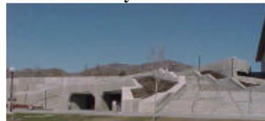
The library addition is a 200,000 s.f., two-story underground facility comprised of mild steel reinforced cast-in-place concrete. The
