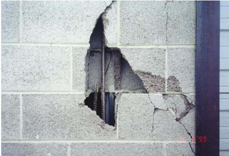
Photo courtesy of Dorian Adams of Reaveley Engineers & Associates. When a truck backed up into this masonry wall, the resulting damage exposed the vertical steel reinforcement. Obviously, the engineer intended the masonry wall to be grouted. Apparently, the contractor had other ideas.
