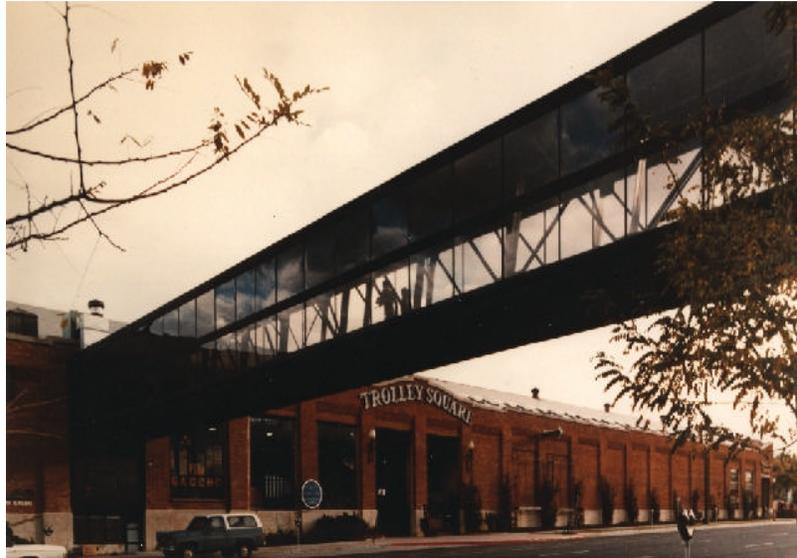
*Bridge over 6<sup>th</sup> South Street to Trolley Square in Salt Lake City Utah. Old smelter truss was analyzed, and retrofitted by Weber Engineering.*
