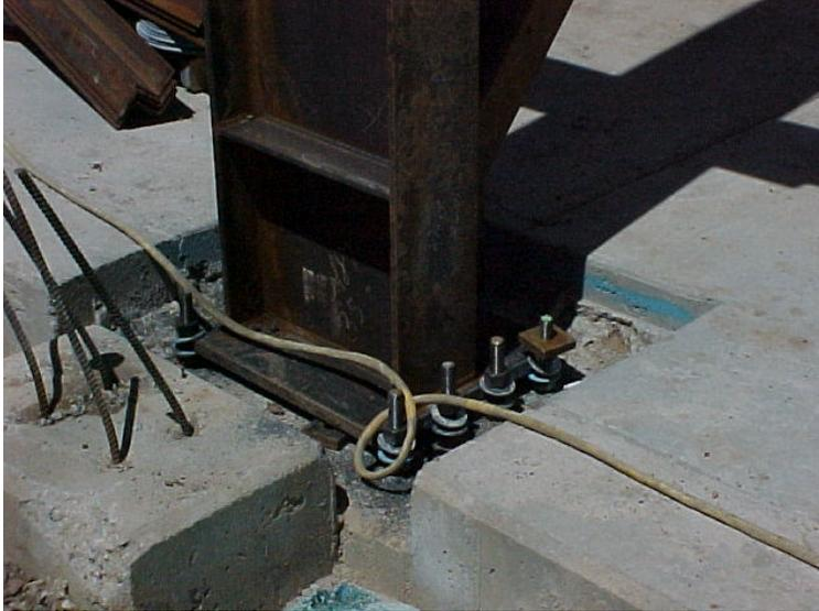
*Steel column to concrete foundation connection has apparently missed the "mark". Submitted by J.M. Williams & Assoc., Inc.*
