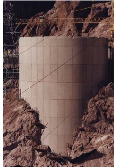
At the Hoover Dam Visitors Center, a 3-D map of the cliff rock face was utilized to cope the precast wall panels to within a 2" dimensional tolerance. This gave the overall appearance of a cylinder projecting from the rock. The precast panels were cantilevered and suspended off of a steel moment frame.
