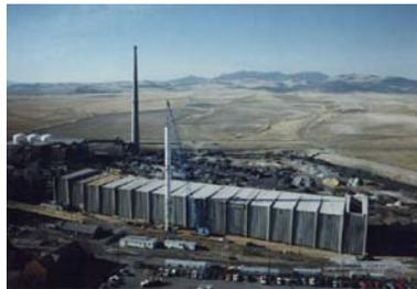
One of our unique precast structures is the ASARCO ore handling facility outside of Helena, Montana. This structure is 105' across by 750' long and has 75' tall wall panels.
