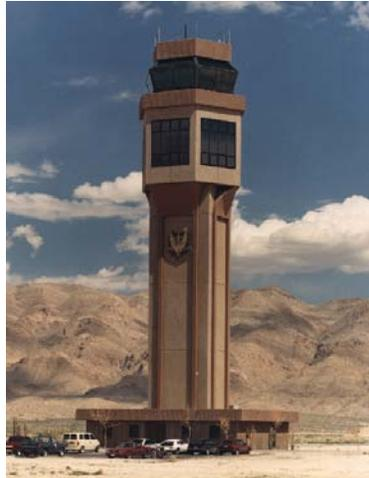
More recently, the Indian Springs air control tower was constructed in Indian Springs Nevada. This Air Force air traffic control tower was designed as an all precast structure.
