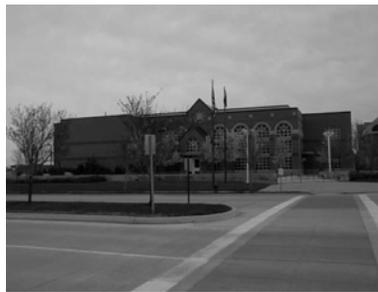
This two-story courthouse and jail has reinforced masonry exterior walls. The floors are framed with open web steel joists, steel deck, and concrete. The columns are of both steel tubular and reinforced concrete sections. This building is complicated with architectural requirements for traffic flow, security, and aesthetics. The basic design is currently under reconstruction in Vernal as the Uintah County Courthouse.
