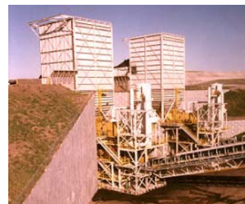
Black Thunder, Wyoming; Semi-Mobile Truck Dump and Crushing Stations
