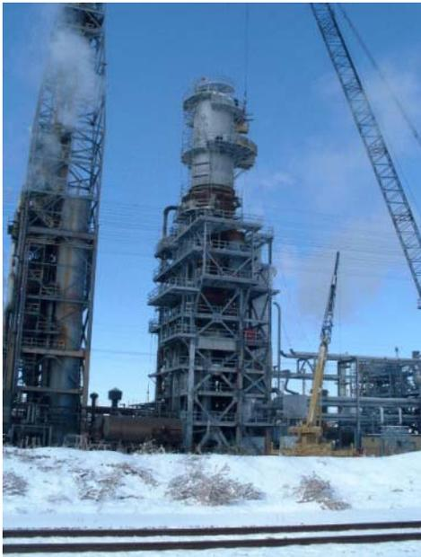
TEC provided structural consulting services to Flying J for the design and fabrication of the MSCC structure. This structure surrounds a new Catalytic Cracker which is currently being installed at the refinery and should be in operation in Apr 2002.
