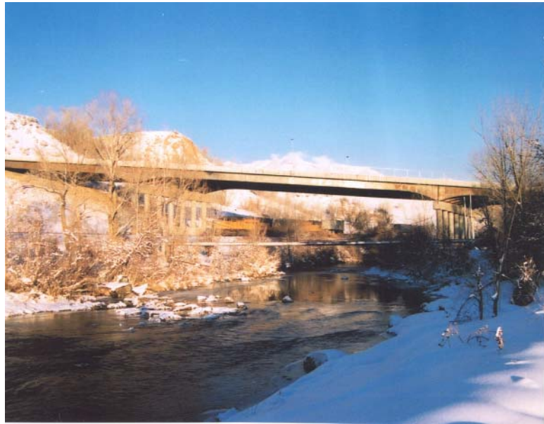
Adams Ave. Bridge link to I-84 south over the Weber River and Union Pacific Railroad tracks in Ogden, Utah, by Ellis & Associates
