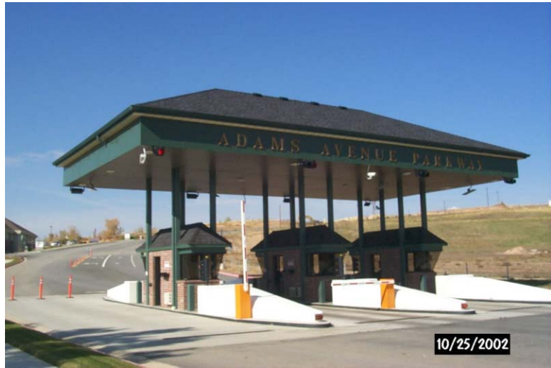
Adams Avenue Parkway Toll Booth Canopy, Washington Terrace, Utah, by Love Engineering, Inc.
