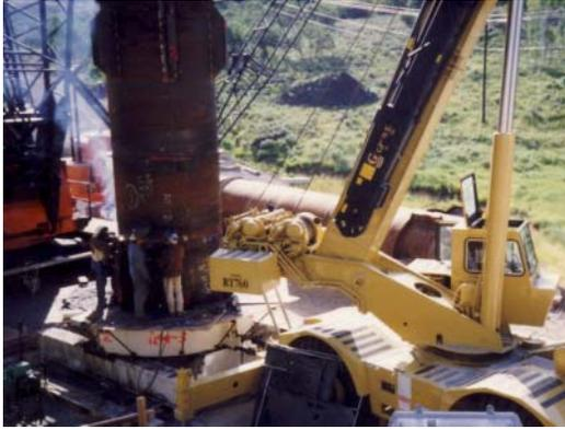
hold the 7.33-foot diameter by 40-foot long steel plate penstock sections as they are lowered by a 300-ton capacity Skyhorse track crane vertically down a 650-foot deep shaft. The clamp holds the penstock sections at ground level while the crane picks and positions the
