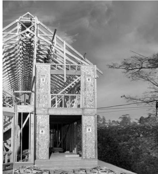
Simpson Strong-Wall shear wall application in a two-story structure, manufactured by Simpson Strong-Tie Co., Inc.
