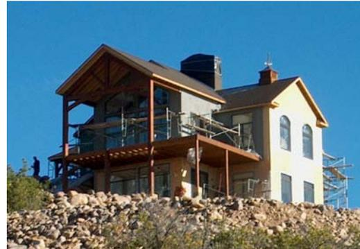
Residence in North Fork is a 4,000 square-foot residence. The design incorporated large rough-cut timber trusses with tall window-filled walls and a floor layout with large open areas. This particular residence included a design adapted to a steeply sloping lot and a roof snow load of 75 psf.
