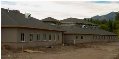
The Ogden Christmas Box House is a shelter facility for children consisting of wood construction. The building consists of two main wings: a dormitory wing and an administration or office wing. The dormitory wing contains a large clerestory area which provides natural light to a large central common area. Large girder trusses are used to create this large common area yet provide support for both the upper and lower roof levels.
