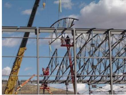
We worked closely with Gem Buildings and Layton Construction to value engineer the design. By utilizing a 15-foot bowstring truss on 10-foot centers we were able to use decking to eliminate the secondary framing. This option provided a significant cost savings to the owner in material and labor costs.
