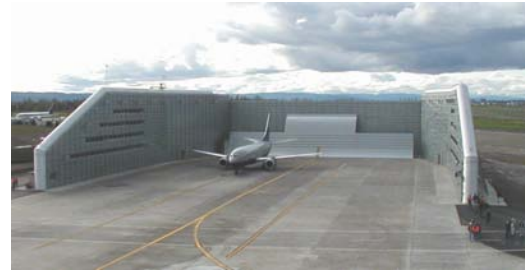
Ground run-up enclosure facility with blast deflector fence, Tampa, Florida
