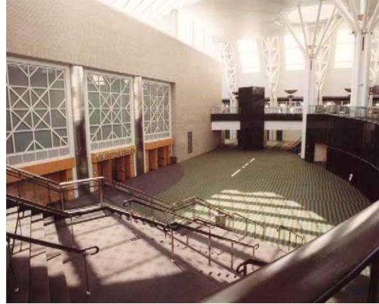
Inside the main entry the **main concourse** of the 1996 expansion is supported by trusses made up of circular steel pipe elements. The trusses were created to open the truss to allow light through the truss into the main concourse. The trusses have a triangular cross section and a sloped profile.
