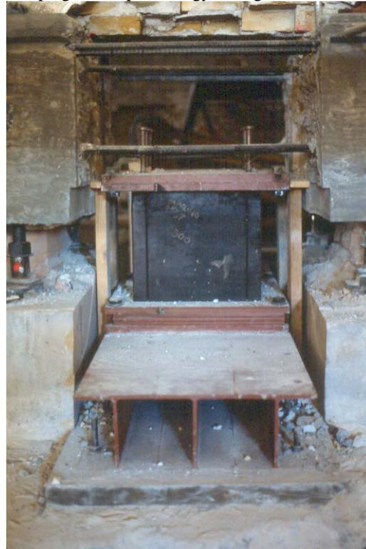
A concrete structural system was added to transfer the loads from the building to the isolators. This load-transfer system consists of concrete beams and a steel grillage. The main elements of the system are described below:
