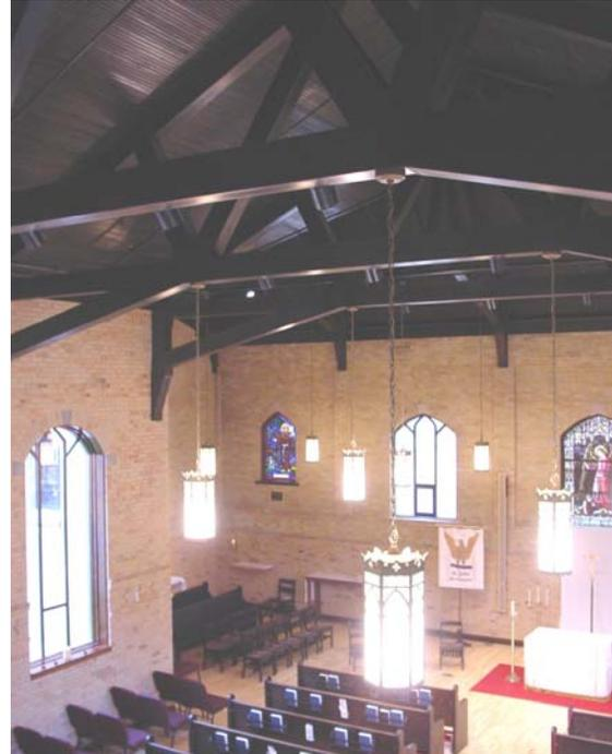
Both, the ceiling in the original chapel and the ceiling in the addition are vaulted ceilings. The architect wanted to remove a portion of the original roof structure to allow the two vaults to merge together as one.
