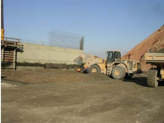
The backfill for the wall was selected and placed carefully. We required that the fill be placed in 6-inch lifts and compacted to 98% of maximum dry density. The concrete fascia wall was 12 inches thick and reinforced with two curtains of rebar that was mostly used to counter the effects of temperature differentials and shrinkage. The fascia wall was designed to resist a small amount of non-accumulating lateral earth pressures. These pressures were the result of backfill
