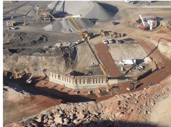
accommodate the close alignment of the crusher, the wall had to be placed vertical within an inch of the crusher frame and no batter was allowed.
