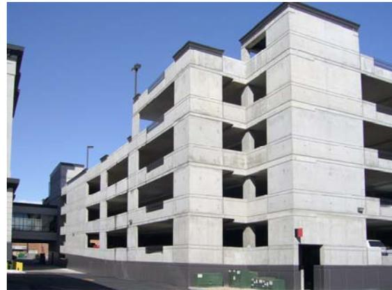
The parking structure layout is a classic 2-bay ramp system. (A bay is referring to a double loaded drive aisle.) Each bay ramps up half a level, a lot like a flight of stairs in a stair well. The structural system however, is a design that is the first of its kind in Utah. Previously, this system has been used in Australia and Texas.
